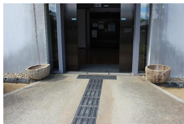
Automatic Door of the Sakagura-kan Reception Building (Width:138cm)
