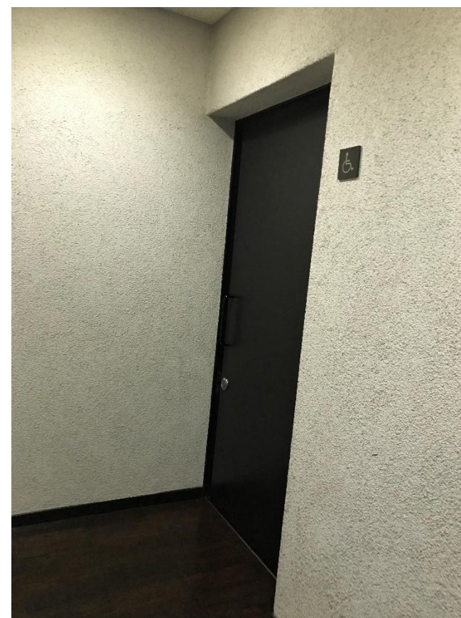
The door of the barrier-free restroom is manual. (Width:87cm)
