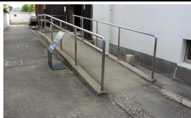
Slope at the Entrance/Exit of Sakagura Building (Width:100cm)
